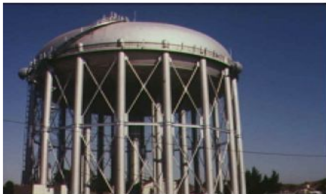
Elevation of retrofitted tank
